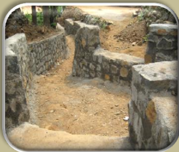
Retaining Wall in Chorawne Village
